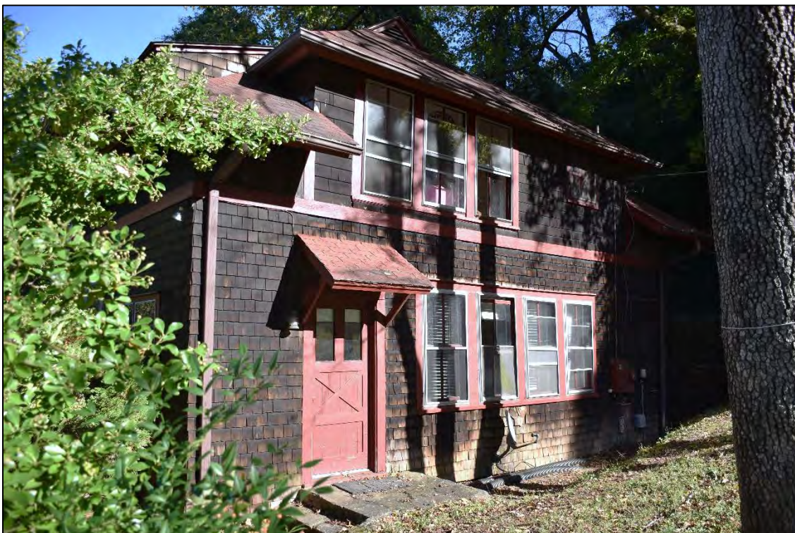
Figure 2.3.7. View of the Washburn House, facing southeast.
