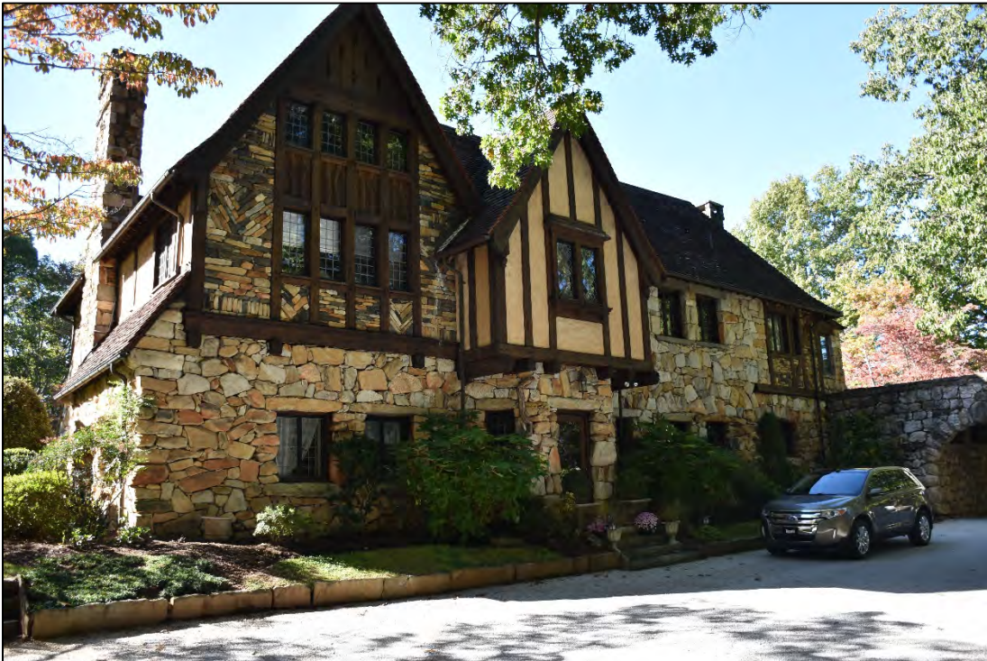
Figure 2.9.19. Lynncote (PL0049), facing northwest.
