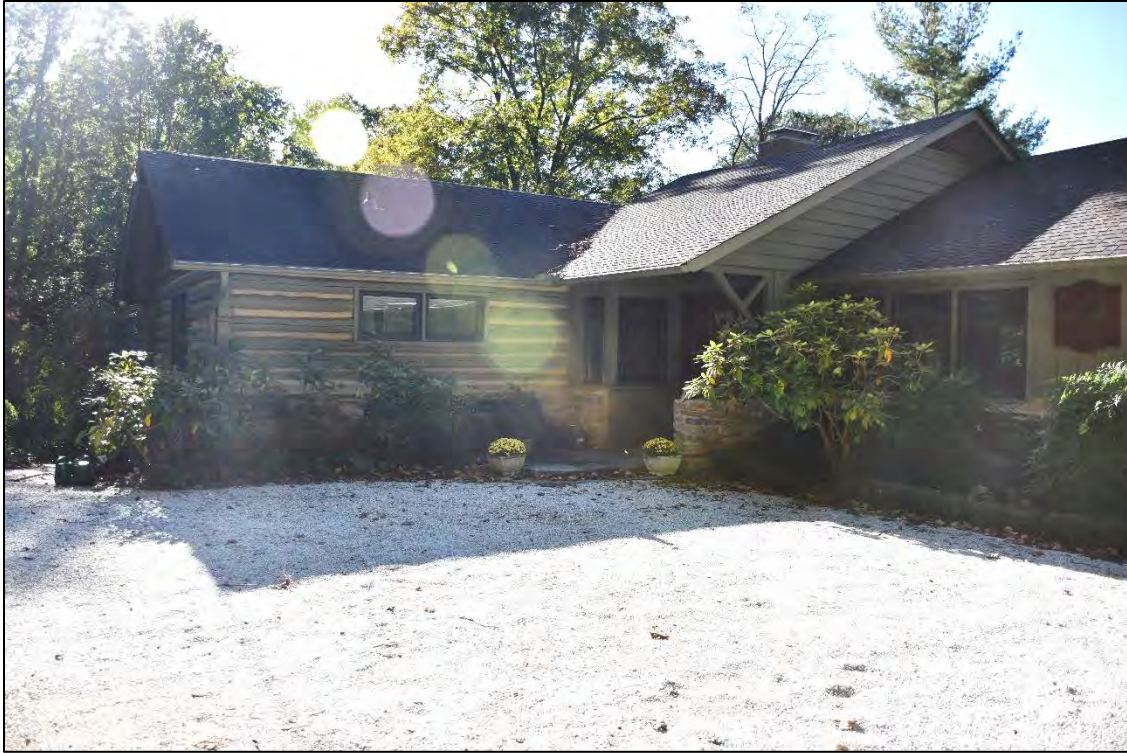
Figure 2.4.4. View of Glencroft, facing west.
