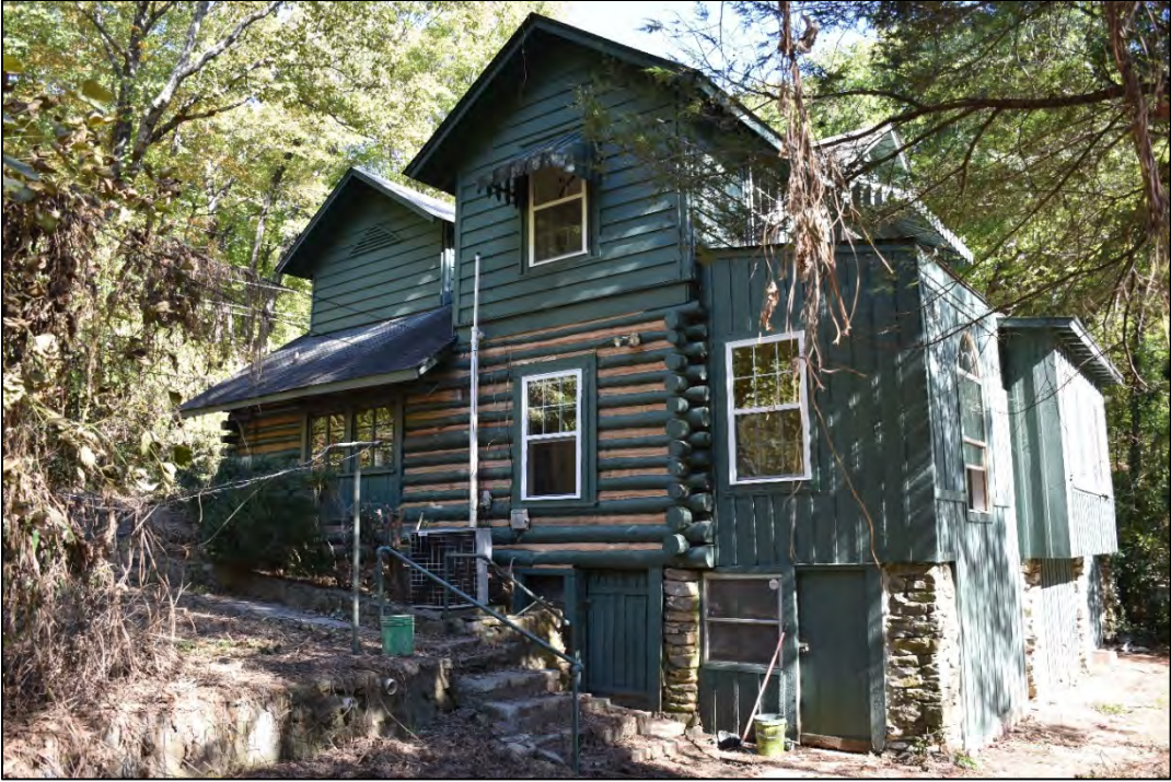
Figure 2.8.3. View of the Uchtmann-Landrum House, facing northeast.
