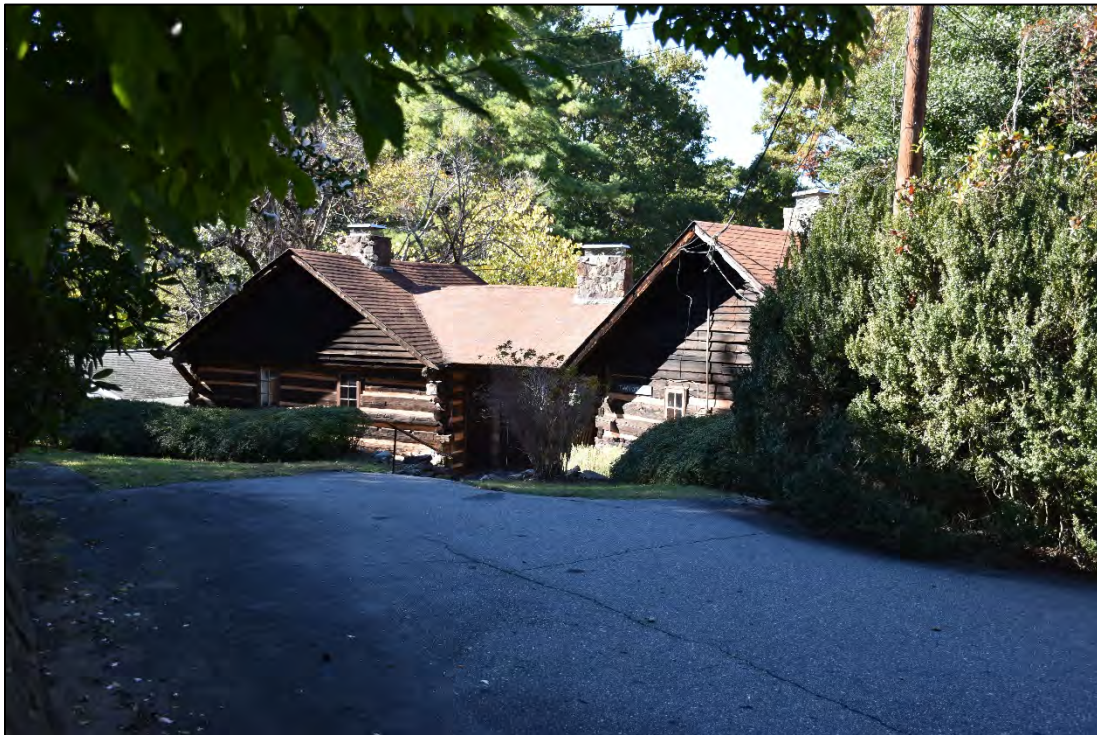
Figure 2.4.15. Twain Cottage at the Pine Crest Inn (PL0006), facing northeast.
