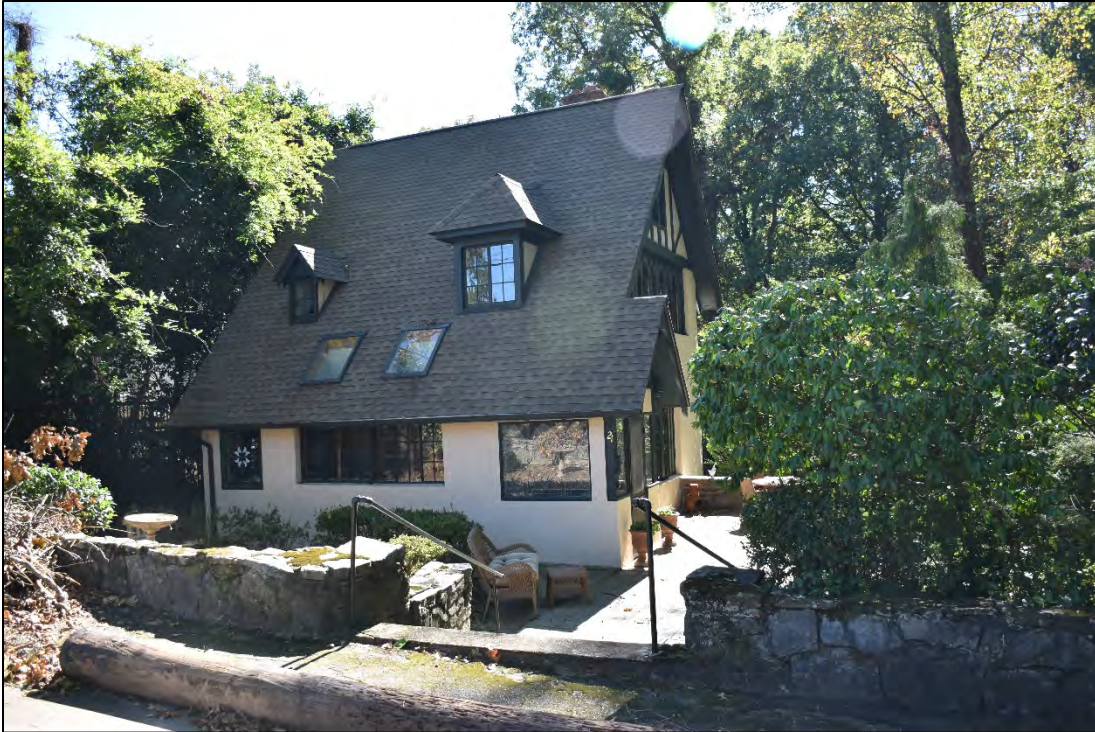
Figure 2.9.20. Woodcarver's House, 331 Melrose Avenue, facing southeast.
