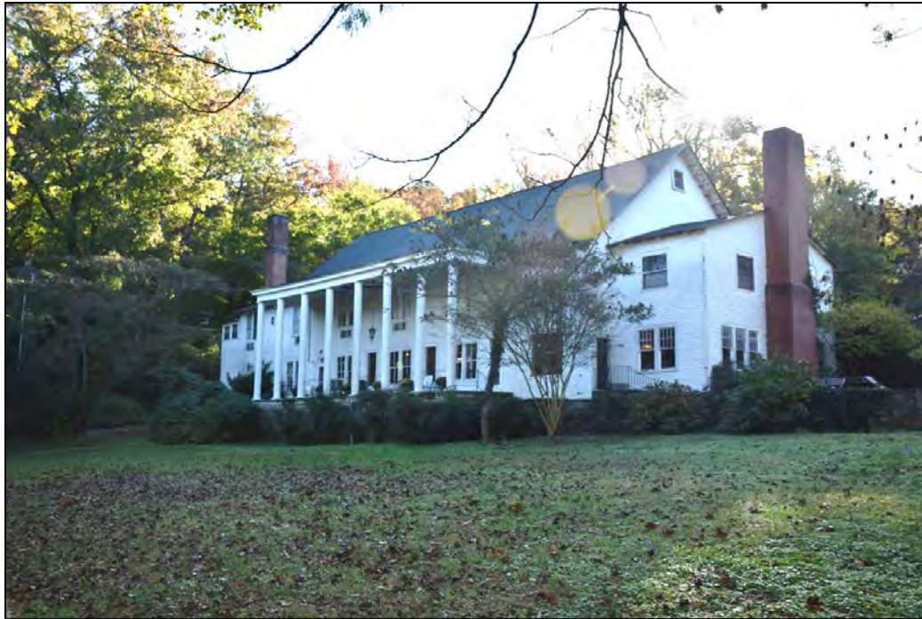
Figure 2.2.3. View of the Mimosa Inn, facing southeast.
