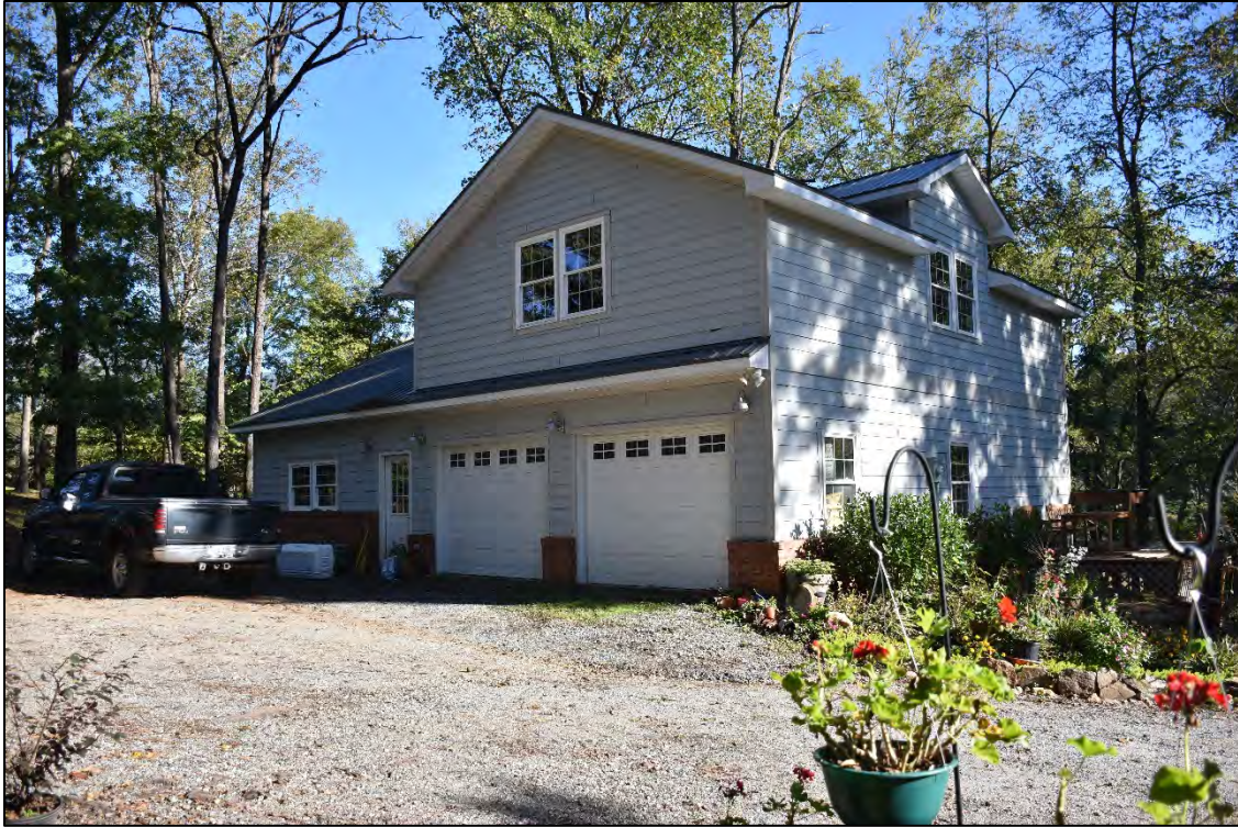
Figure 2.1.17. View of modern garage, Sidney Lanier House, facing northeast.
