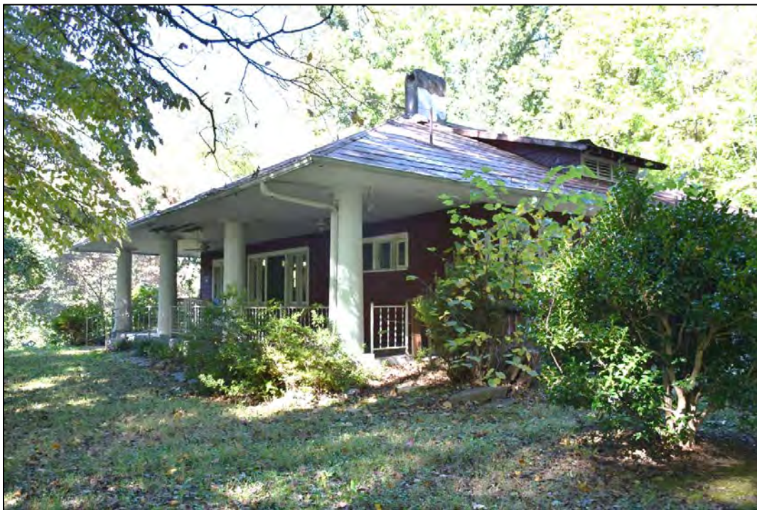
Figure 2.7.3. View of Over the Way, facing north.
