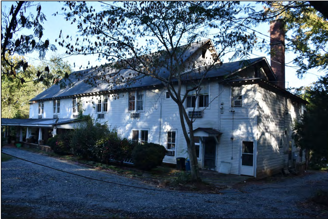
Figure 2.2.8. View of the Mimosa Inn, rear elevation, facing northwest.
