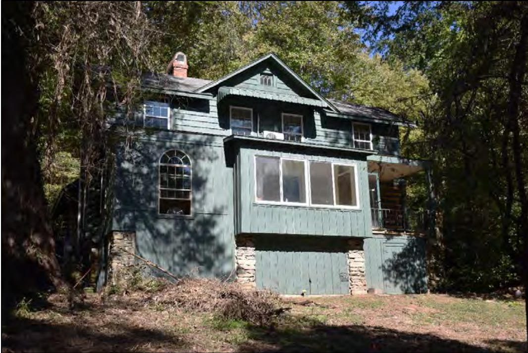
Figure 2.8.2. View of the Uchtmann-Landrum House, facing northeast.
