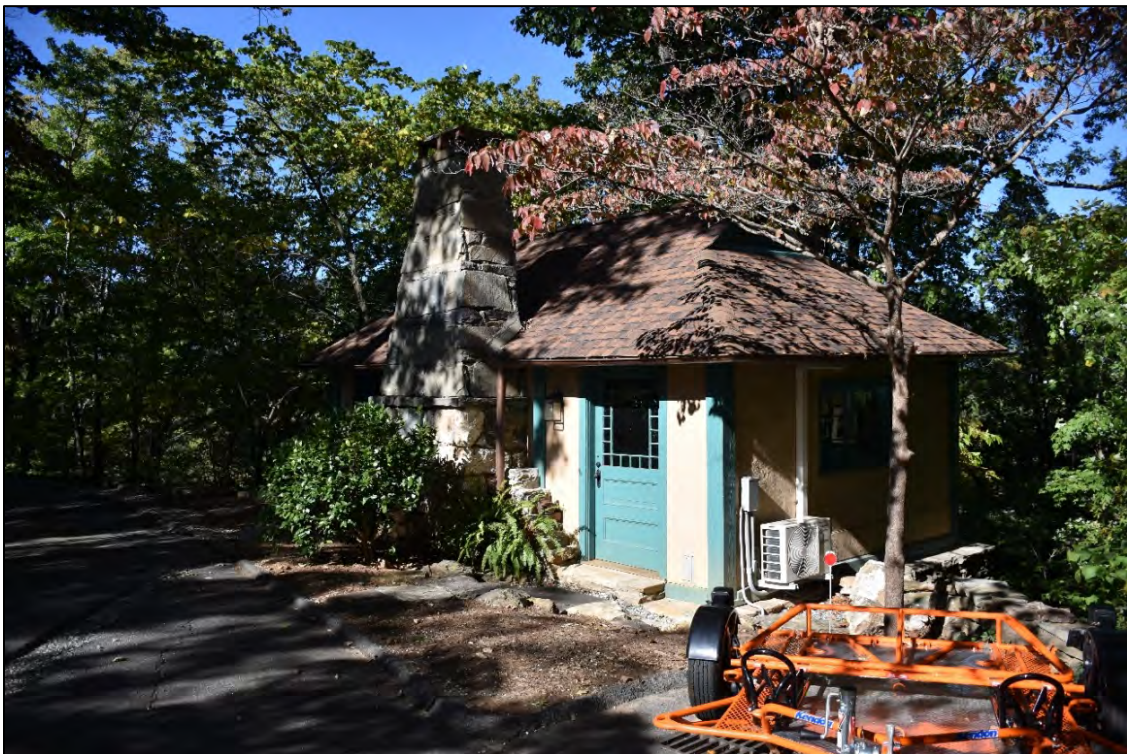
Figure 2.6.3. View of the Workshop building at Lynncote, facing north.
