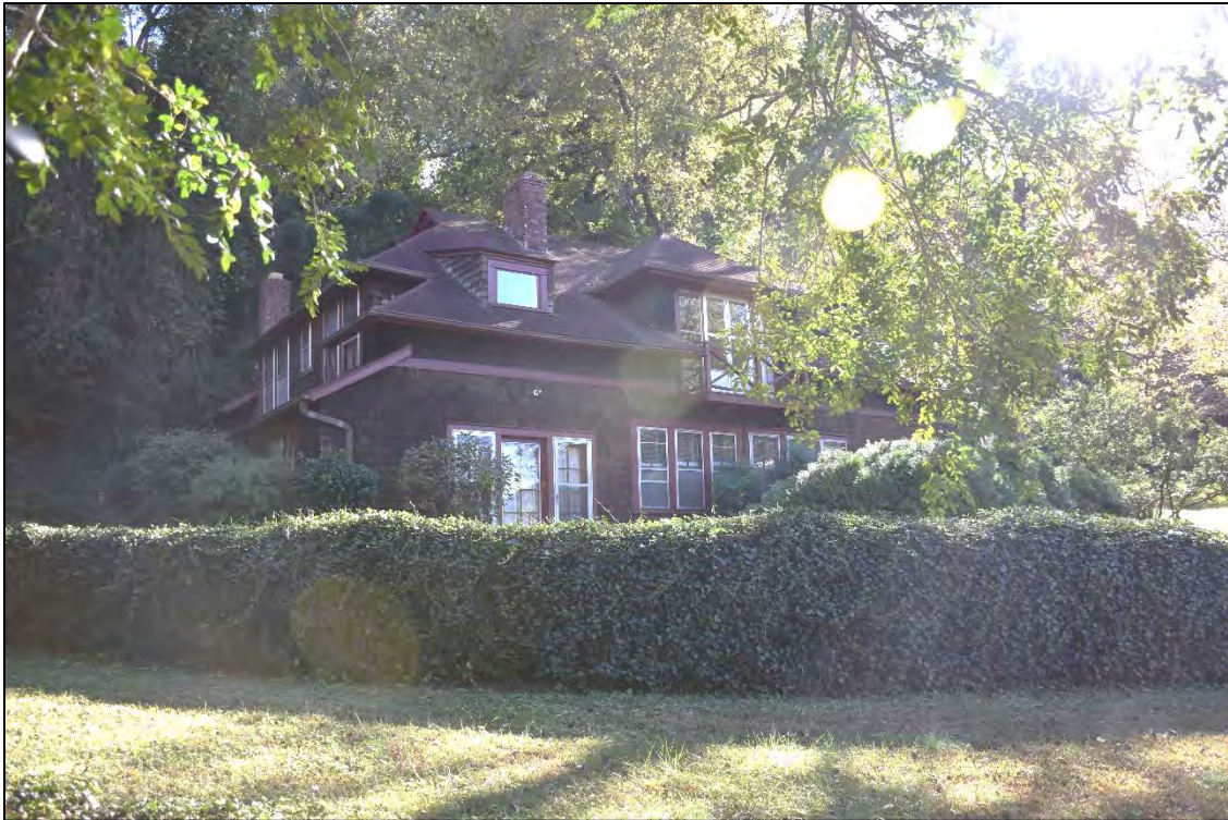
Figure 2.3.2. View of the Washburn House, facing southwest.
