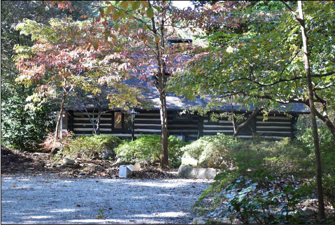
Figure 2.4.16. House at 123 Thousand Pines Lane, facing southwest.
