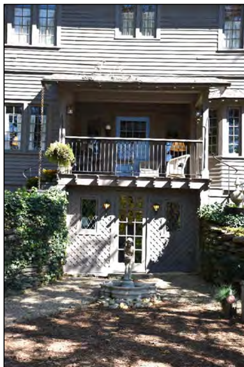
Figure 2.9.3. Mostly Hall, main entrance detail, facing northeast.
