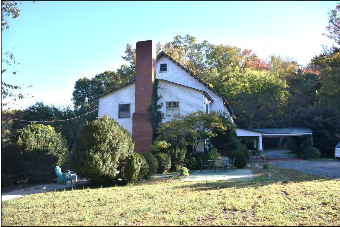
Figure 2.2.5. View of the Mimosa Inn, facing east.
