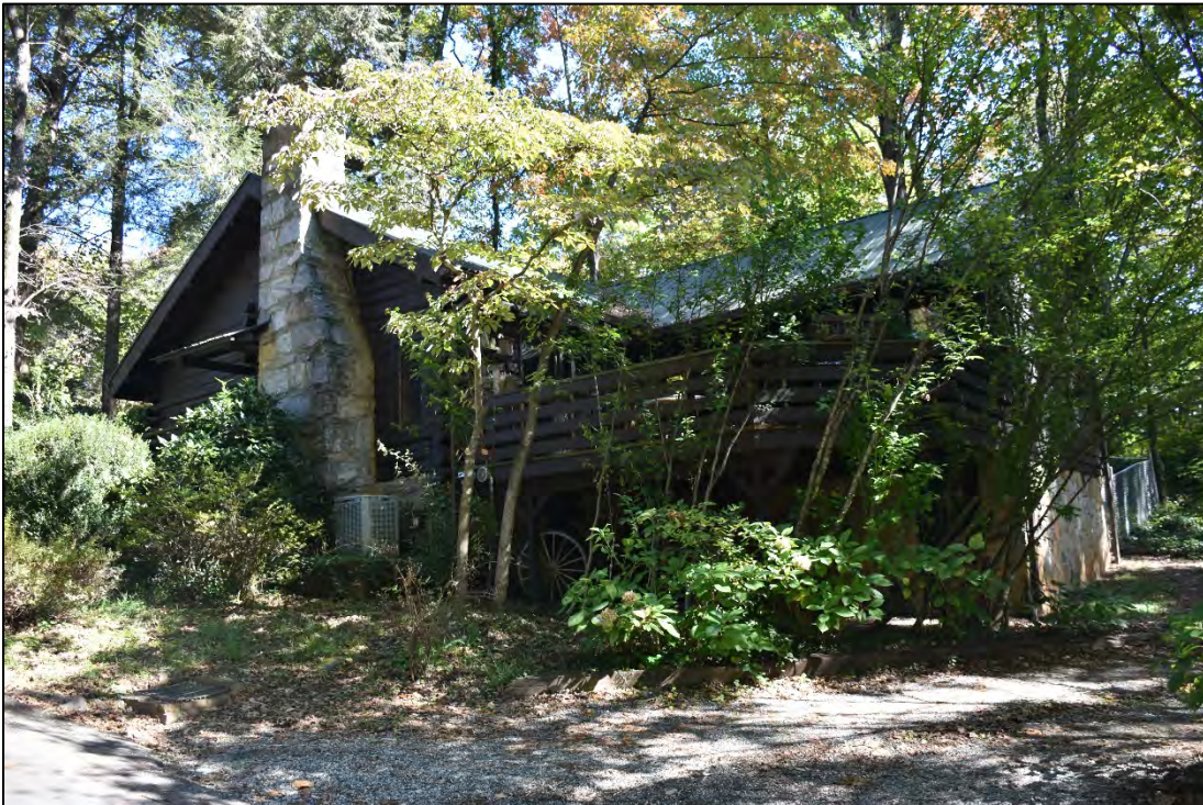
Figure 2.8.15. House at 386 Melrose Avenue, facing northwest.
