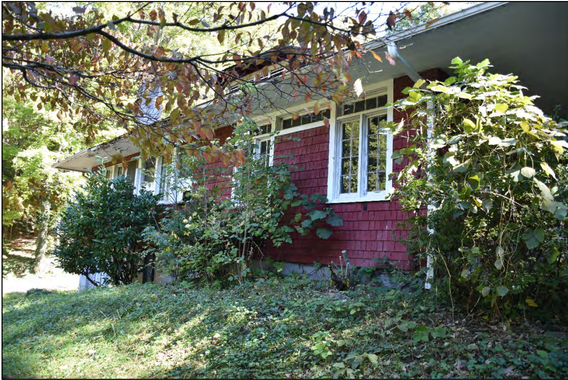
Figure 2.7.8. View of Over the Way, facing east.
