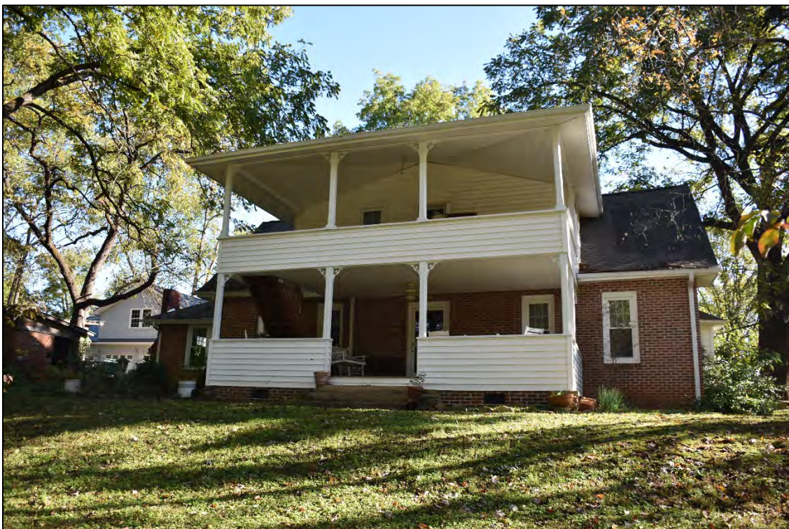
Figure 2.1.5. View of Sidney Lanier House, facing east.
