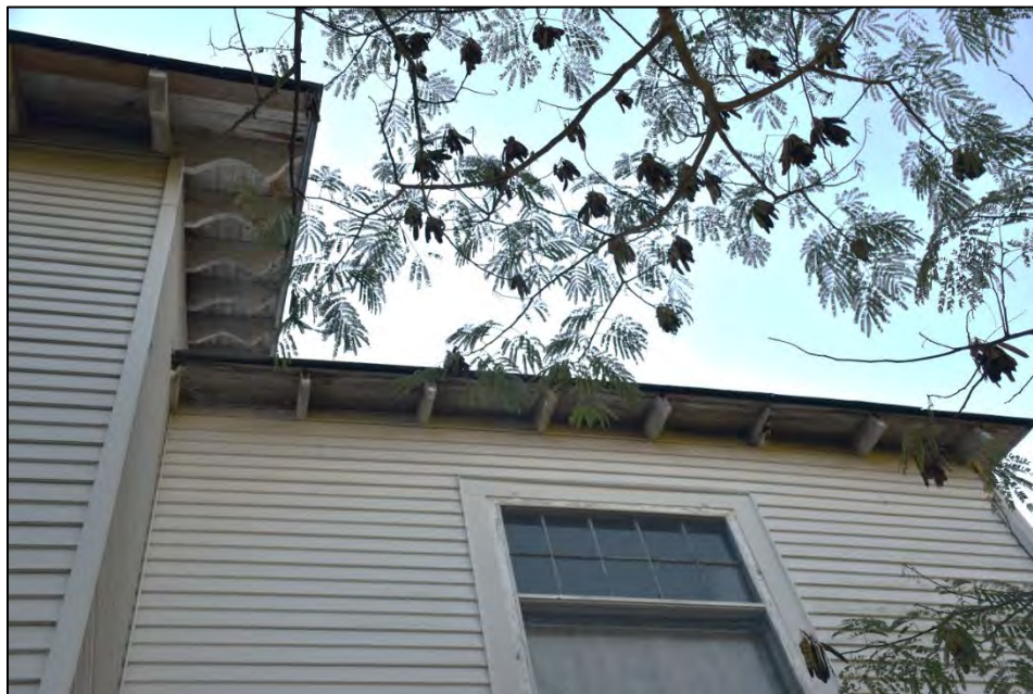
Figure 2.2.11. View of the Mimosa Inn, eave brackets, facing south.
