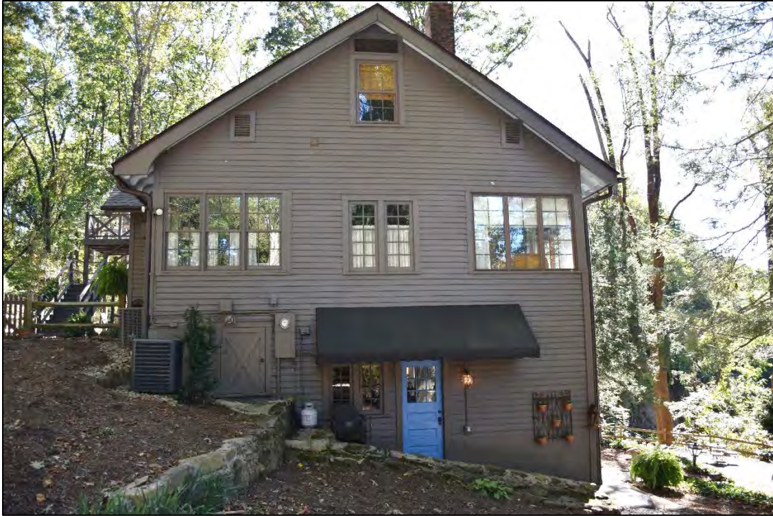
Figure 2.9.8. View of Mostly Hall, facing southeast.
