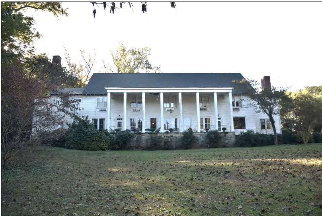
Figure 2.2.1. View of the Mimosa Inn, facing south.
