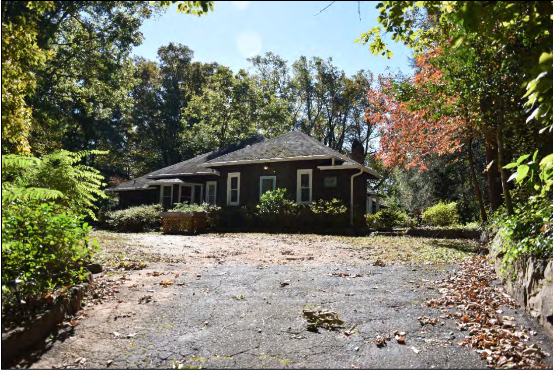
Figure 2.3.13. House at 247 Melrose Circle, facing south.
