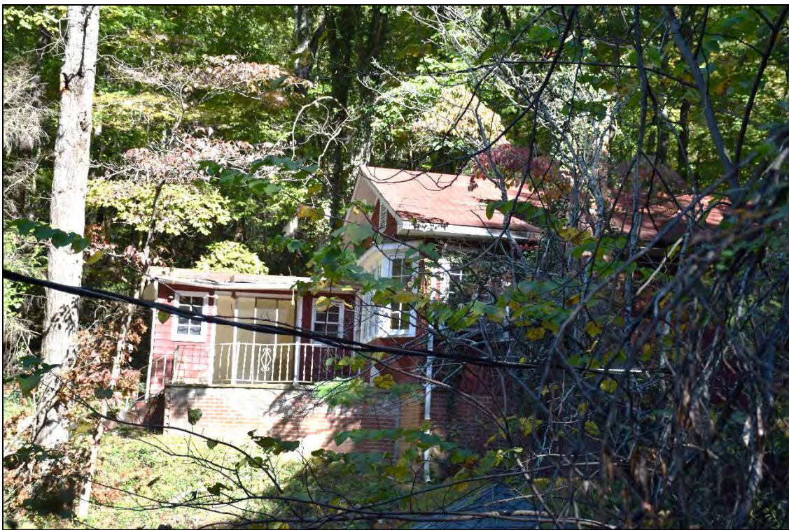
Figure 2.7.11. View of mid-twentieth-century guest house, Over the Way, facing northeast.
