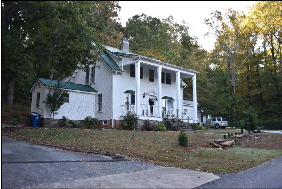
Figure 2.2.29. House at 115 Mimosa Inn Drive, facing southeast.
