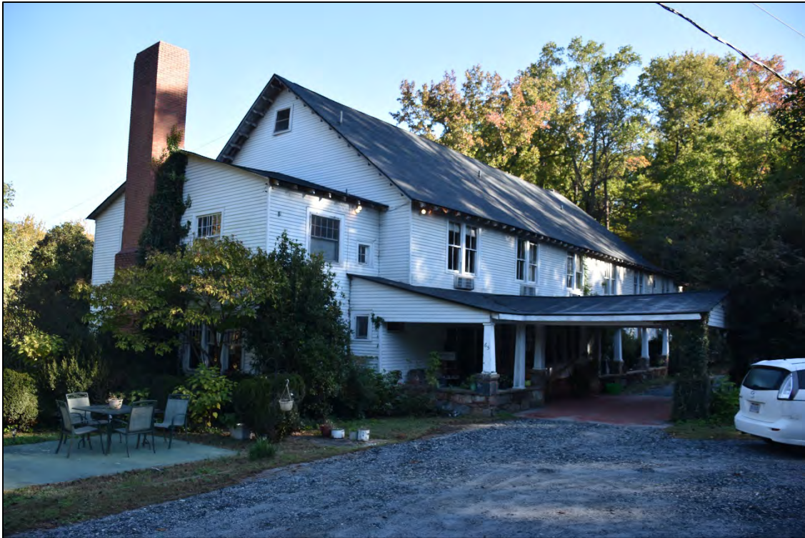
Figure 2.2.6. View of the Mimosa Inn, facing northeast.
