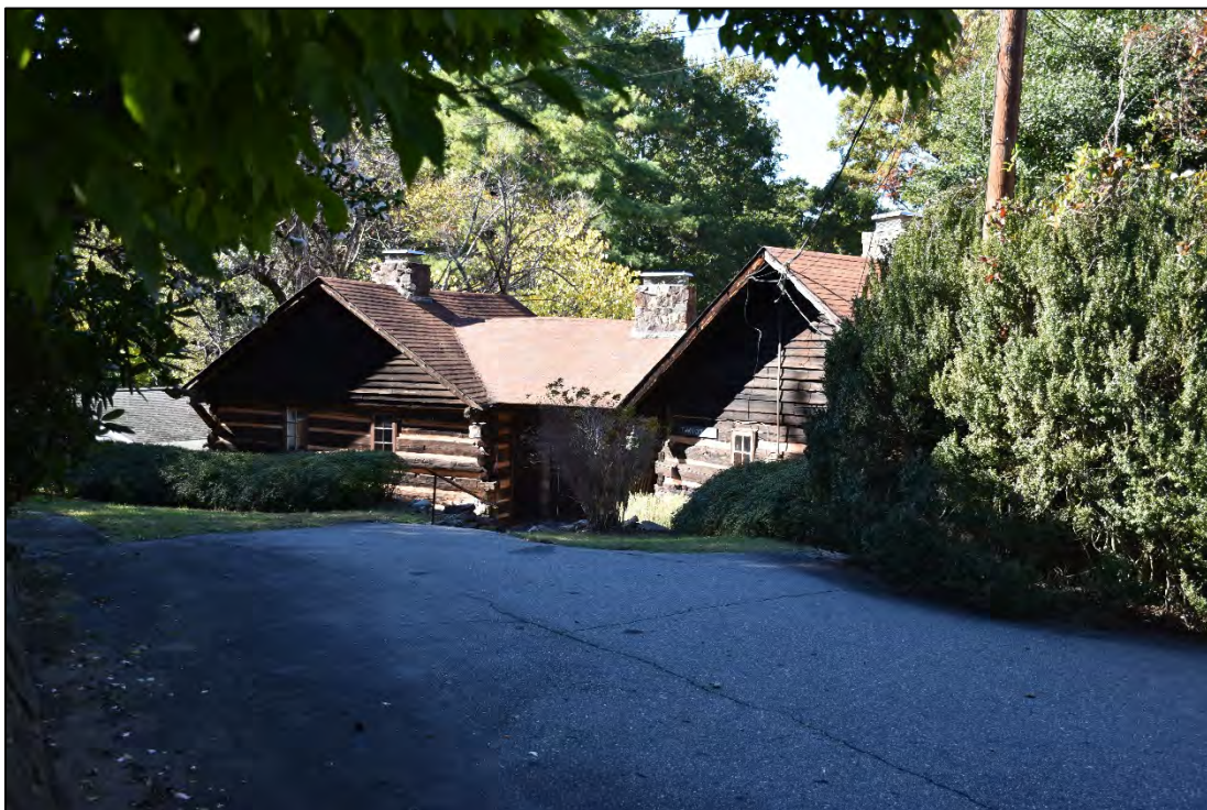
Figure 2.8.13. Twain Cottage at the Pine Crest Inn (PL0006), facing northeast.
