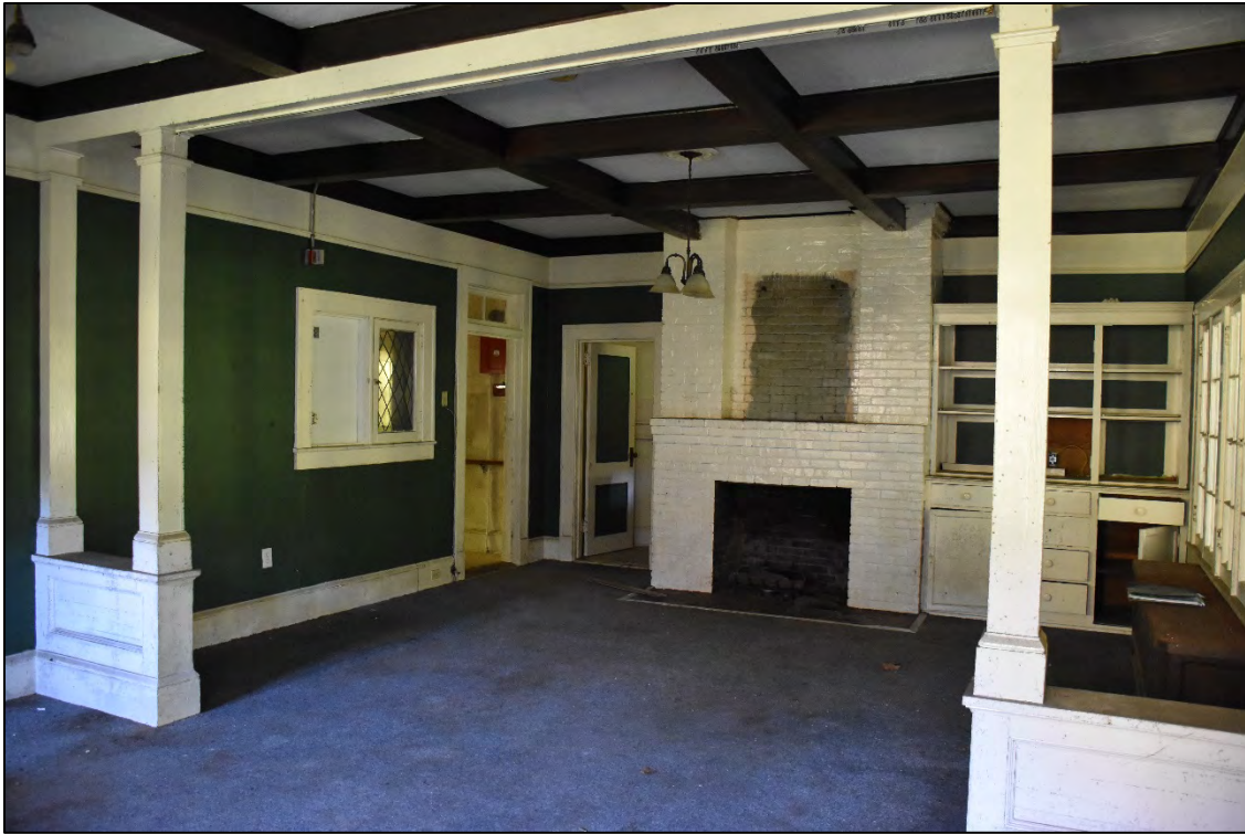
Figure 2.7.9. View of Over the Way, interior, facing northwest.
