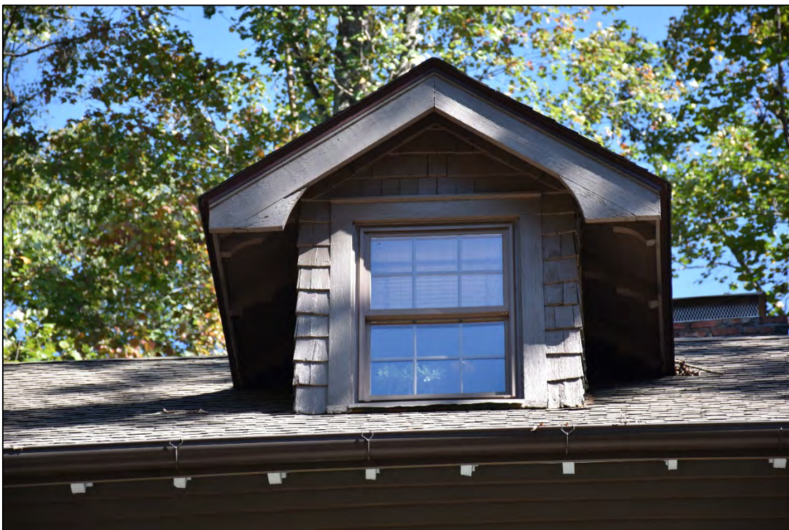
Figure 2.9.5. Mostly Hall, dormer detail, facing northeast.
