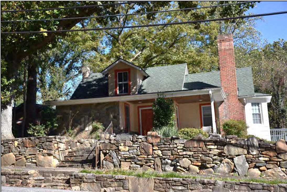
Figure 2.7.26. House at 238 Grady Avenue, northeast.
