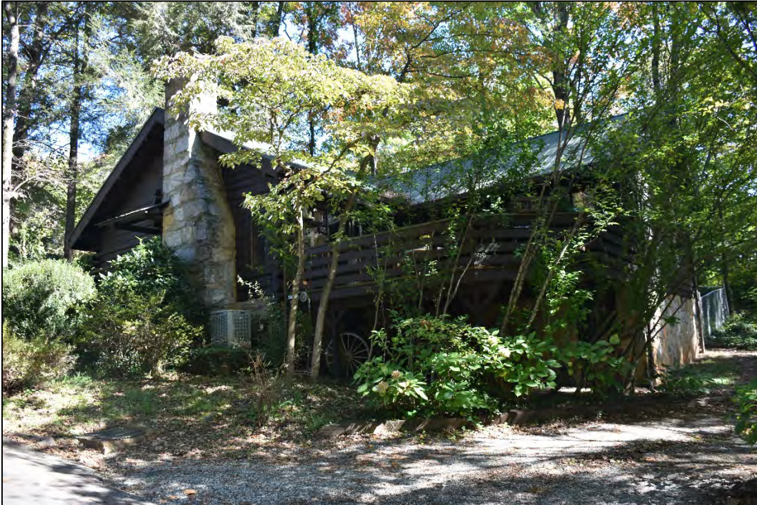
Figure 2.4.17. House at 386 Melrose Avenue, facing northwest.
