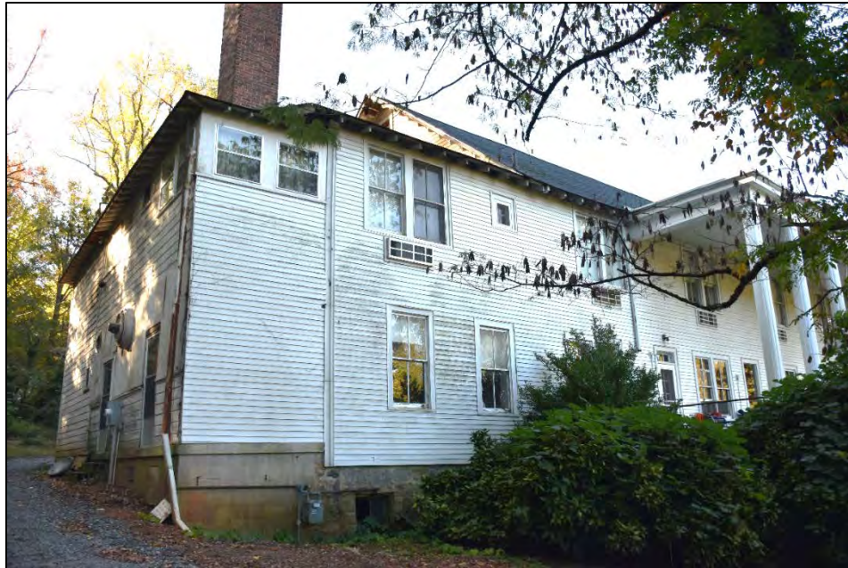
Figure 2.2.10. View of the Mimosa Inn, facing southwest.
