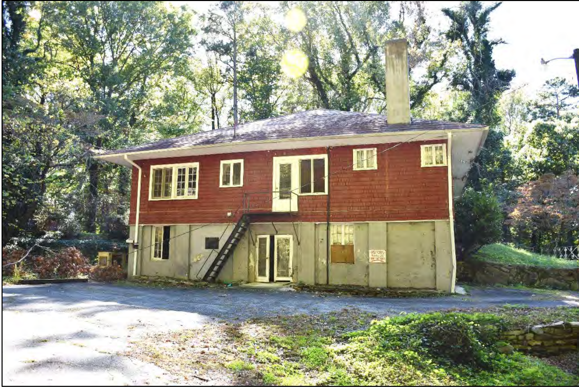
Figure 2.7.6. View of Over the Way, facing southwest.
