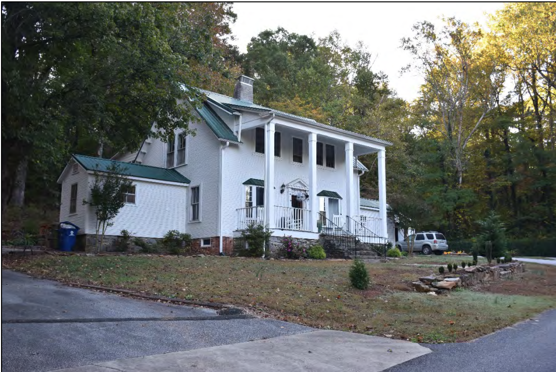
Figure 2.1.22. House at 115 Mimosa Inn Drive, facing southeast.
