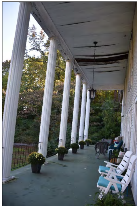
Figure 2.2.4. View of the Mimosa Inn, porch and columns, facing east.
