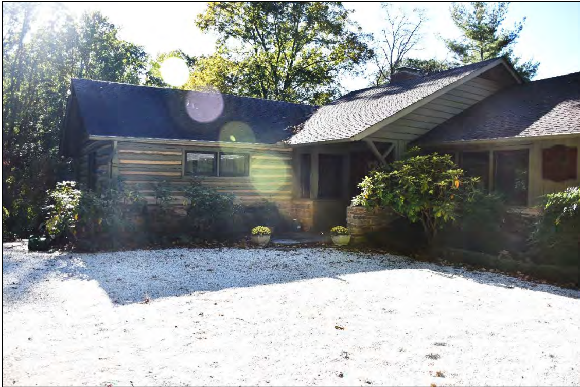
Figure 2.8.12. Glencroft (PL0307), facing west.
