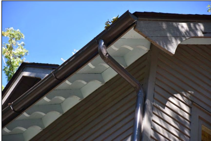
Figure 2.9.10. Mostly Hall, eave bracket detail, facing north.
