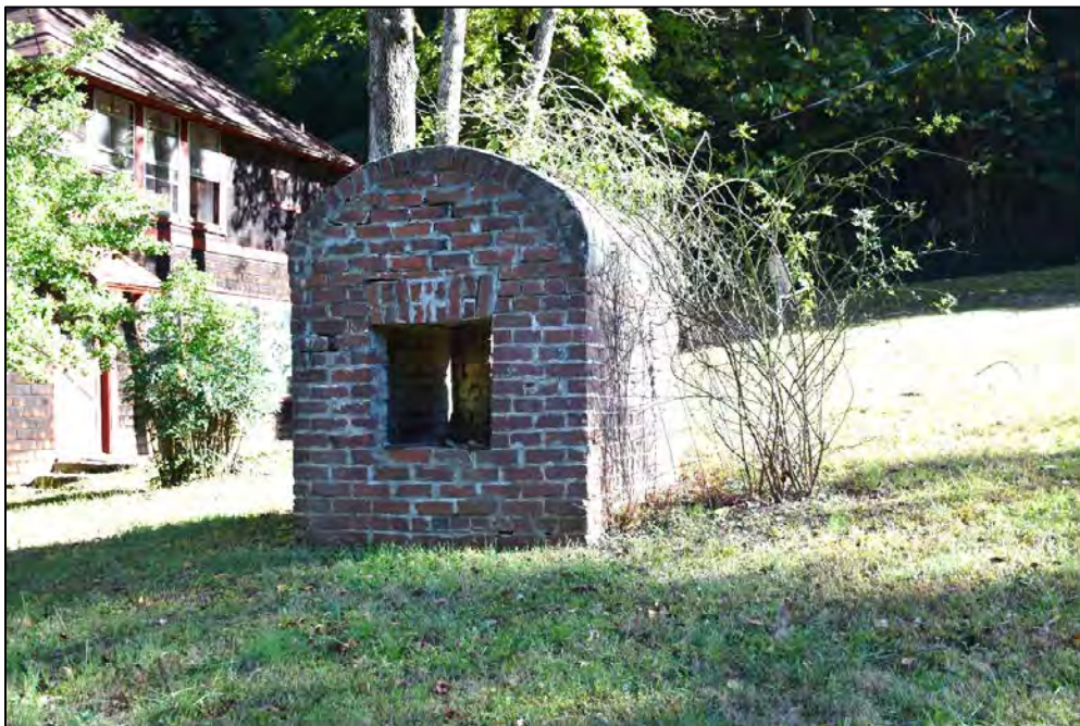
Figure 2.3.9. View of the Washburn House, outdoor oven, facing southeast.
