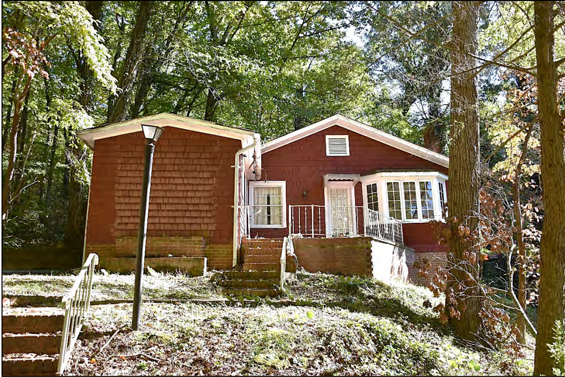
Figure 2.7.12. View of mid-twentieth-century guest house, Over the Way, facing east.
