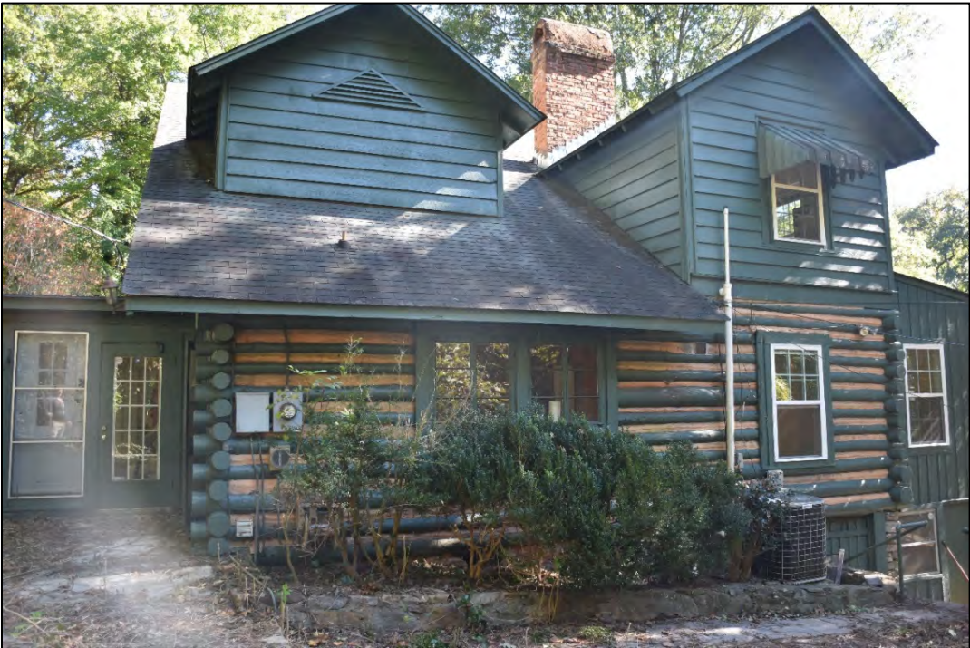
Figure 2.8.4. View of the Uchtmann-Landrum House, facing east.
