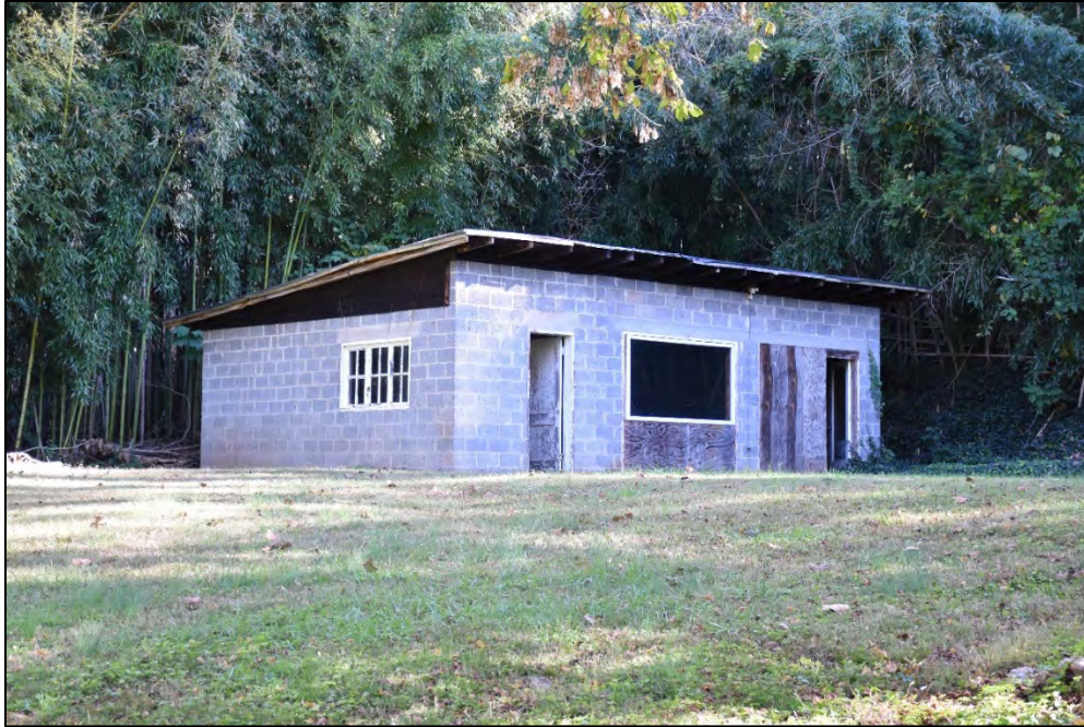
Figure 2.3.8. View of the Washburn House, garage, facing east.
