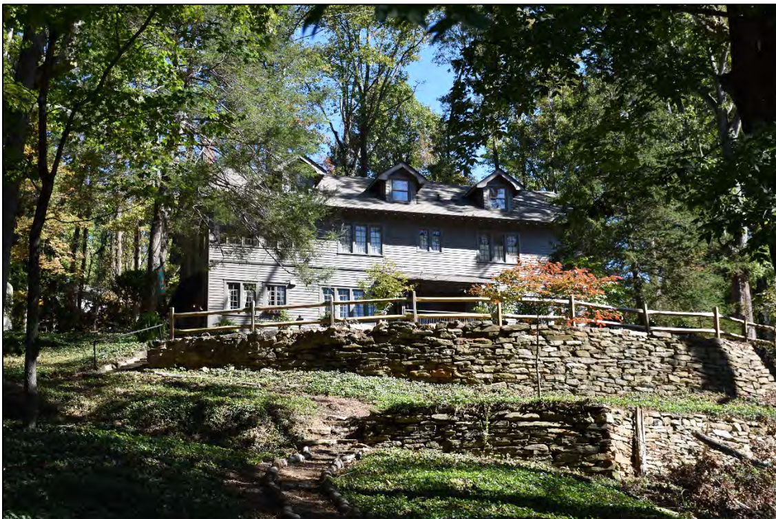
Figure 2.9.1. View of Mostly Hall, facing east.
