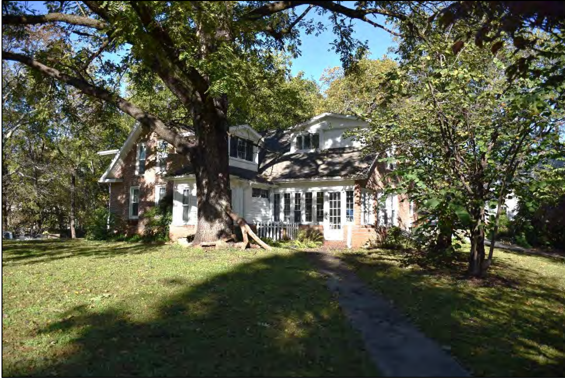
Figure 2.1.6. View of the Sidney Lanier House, facing northwest.
