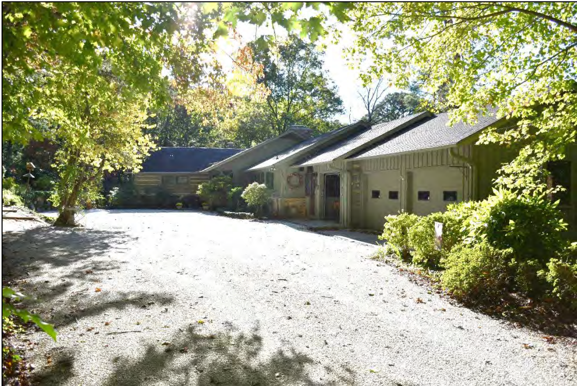
Figure 2.4.1. View of Glencroft, facing west.
